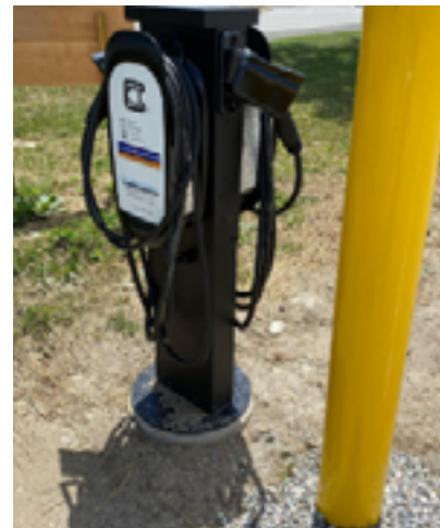
An example of a pedestal-mounted Level 2 charger.
